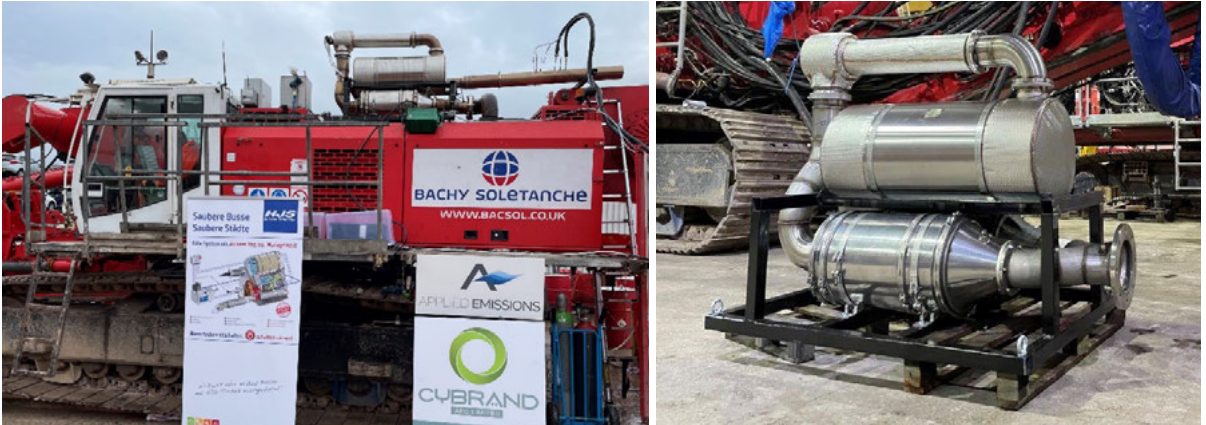
Figure 16: Piling Rig BG 40 – UK
