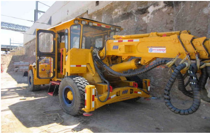
Figure 18: Amtrak Tunnel Project, Long Island City, NY
